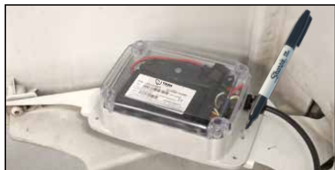
Figure 2: Mark drilling template
